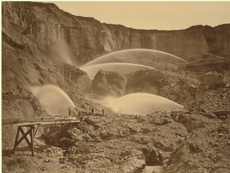
BOX 33.4 FIGURE 2 Water cannons at Malakoff Diggins used to erode sediment into sluice boxes for gold recovery. Mine tailings flowed into the South Yuba River. Photo: Courtesy of the Bancroft Library, UC Berkeley.
